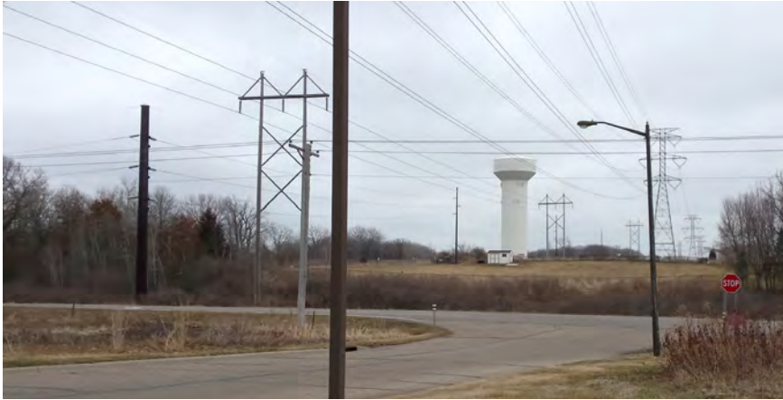
Looking from the St. Thomas Becket parking lot to the east, the Highline corridor crossing of TH3 / S. Robert Trail sets up topographically well for a bridge, but the numerous power poles and lines provide a challenge to work around.
