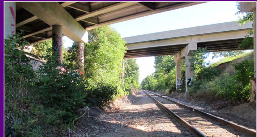
Railroad underpass of Hwy 52
