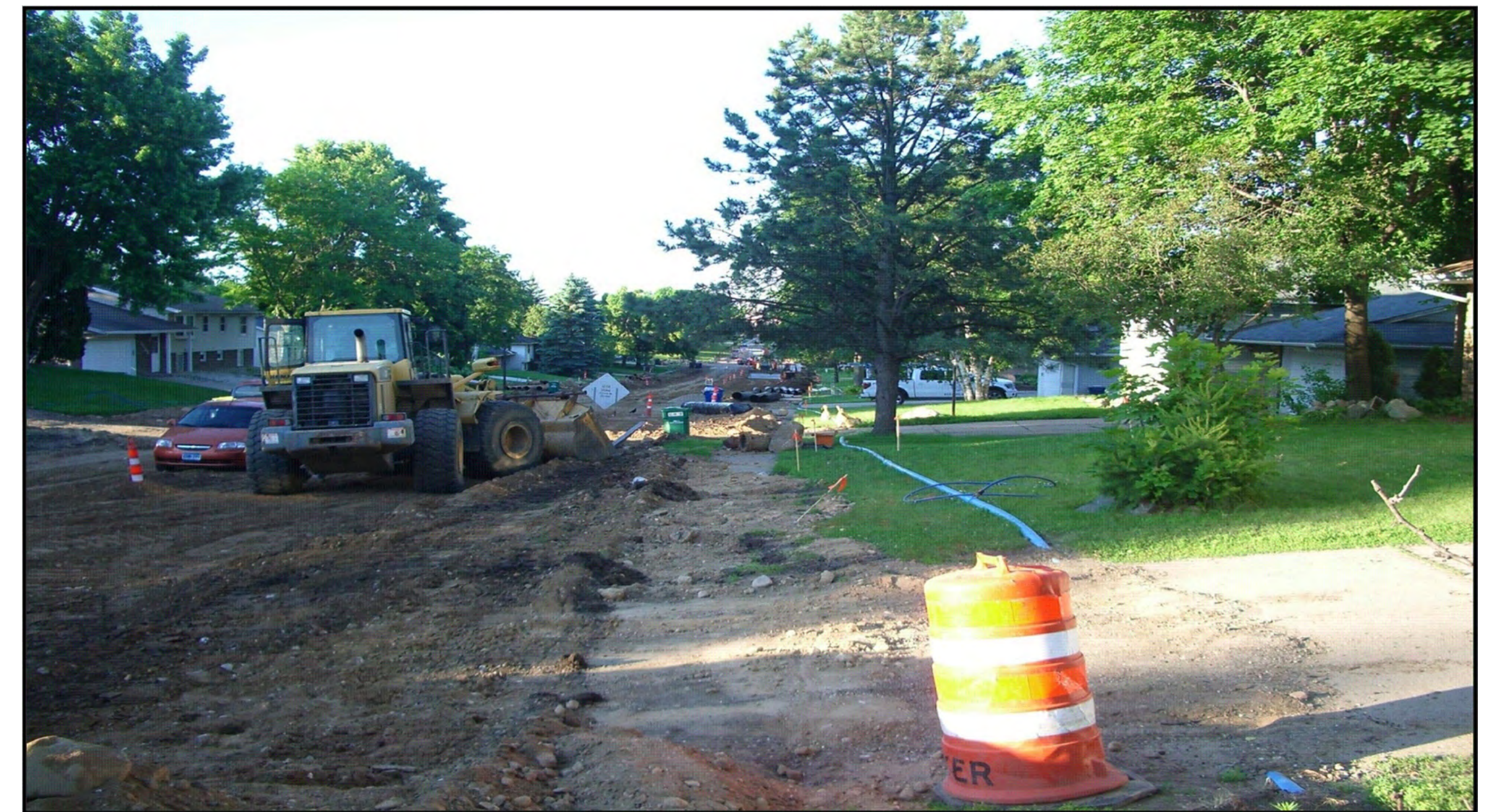
Temporary Water Service
