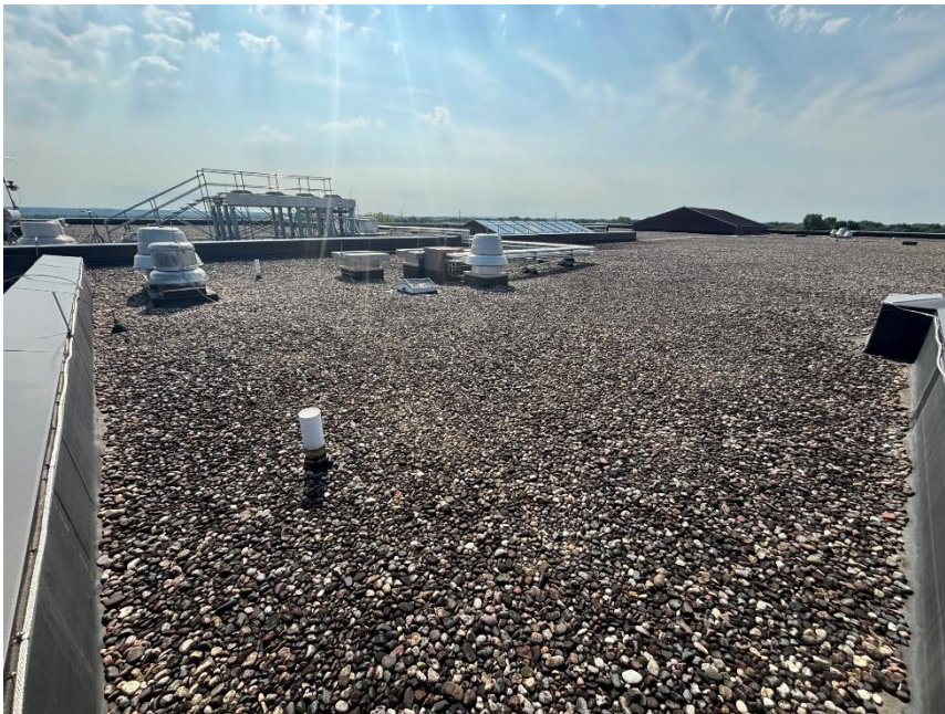
Figure 5 - Rooftop towards Vertical Penetration
