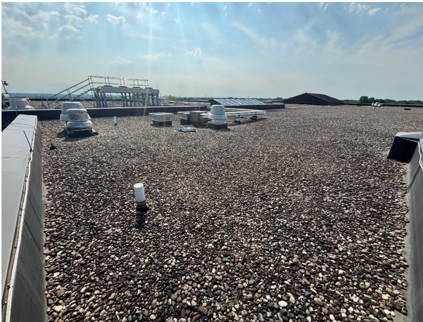
Figure 5 - Rooftop towards Vertical Penetration
