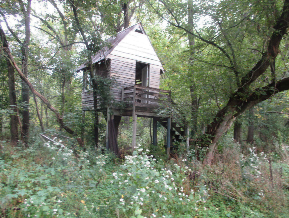
Photograph 8 09/03/26 Subject Tree house NW of barn
