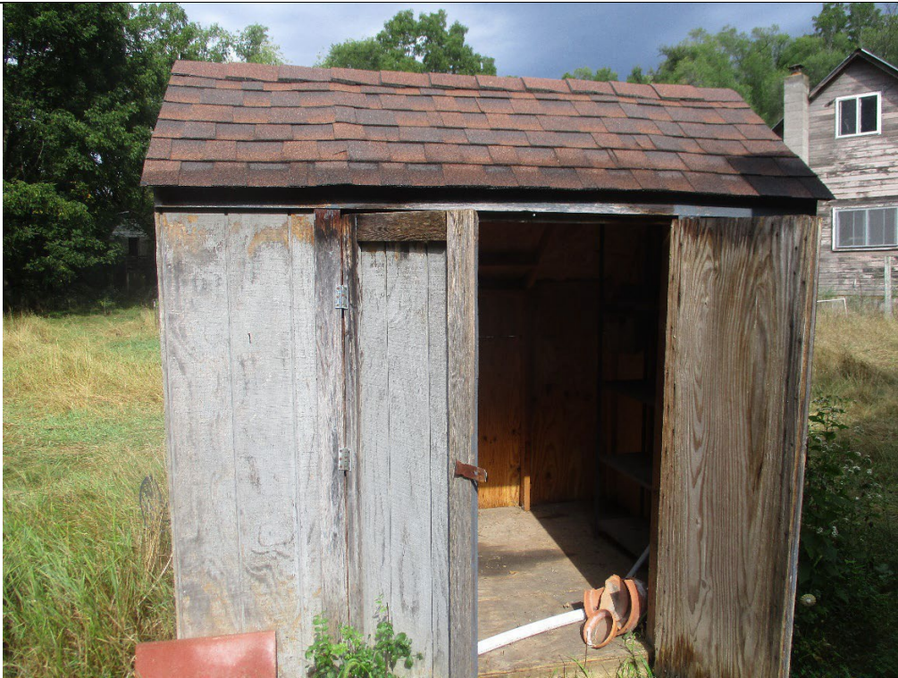
Photograph 7 09/03/26 Subject: Small shed NW of trailer house
