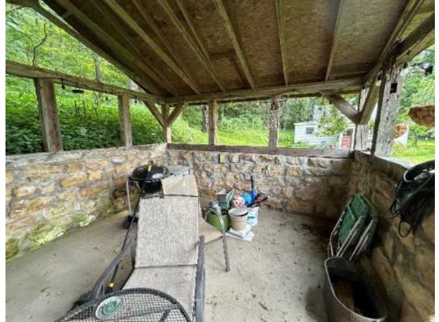
Interior of the grilling structure
