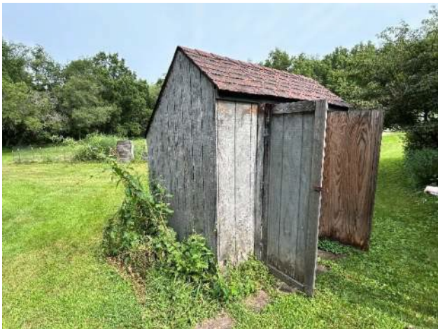
Wood shed located on the Property
