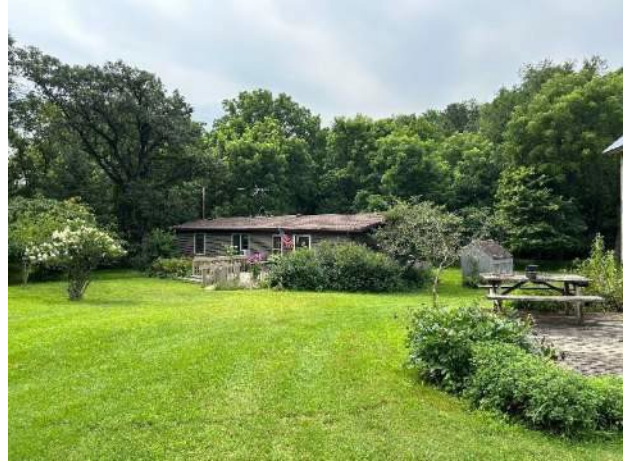
Mobile Home located on the Southern portion of the Property
