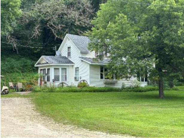
Main House located on the Property
