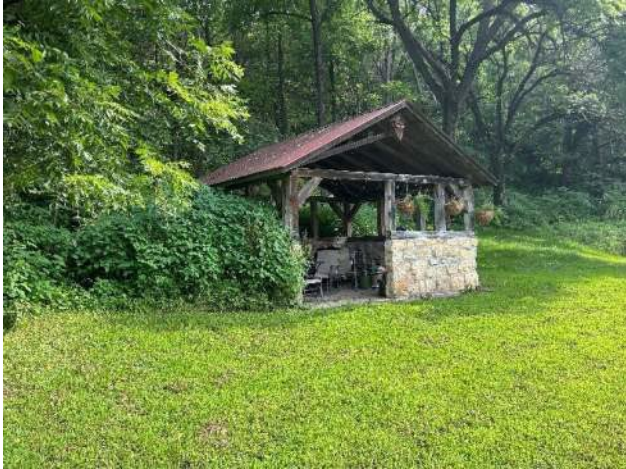
Grilling structure located on the Property
