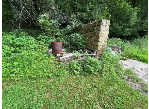
Old foundation with miscellaneous wood.
