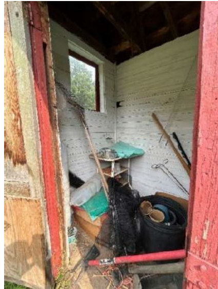
Interior of the red shed.
