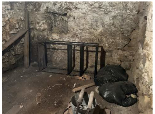
Basement of the main house
