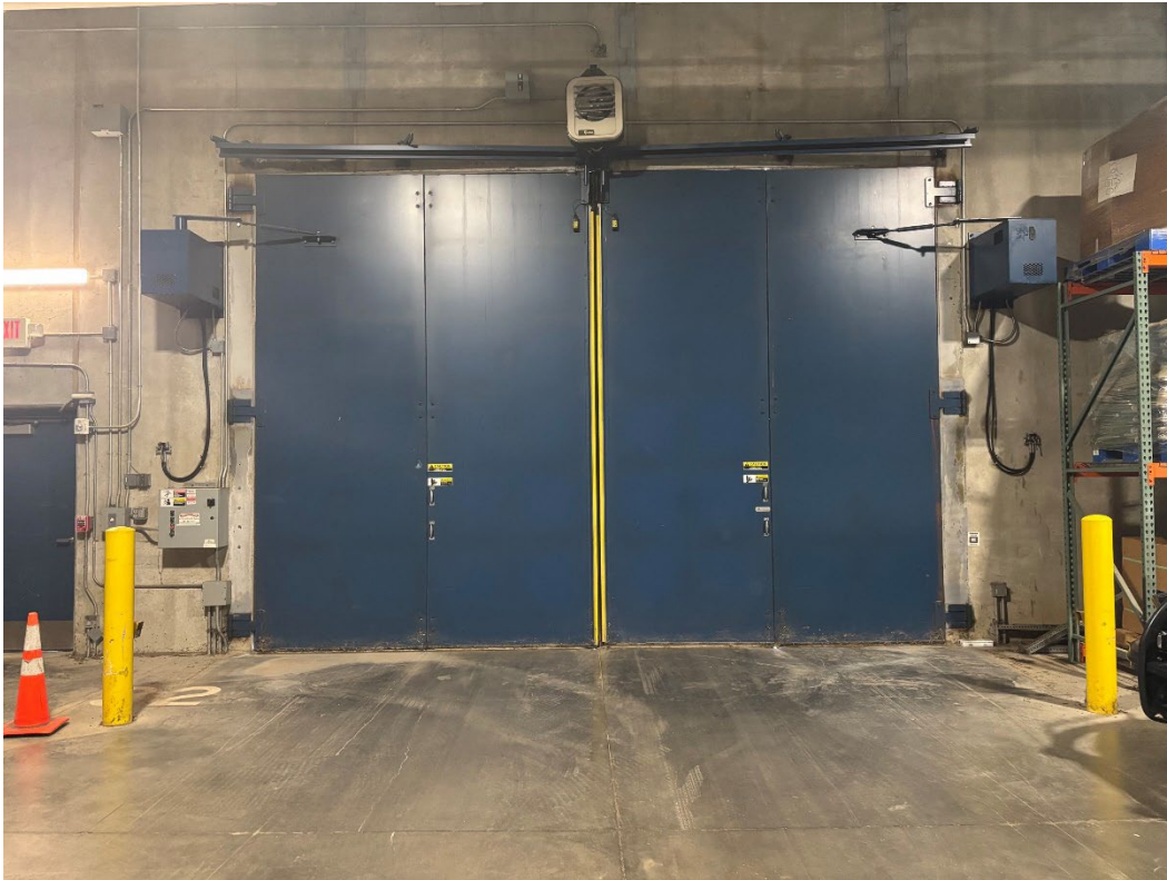
Figure 3 - Southwest Interior Door View
