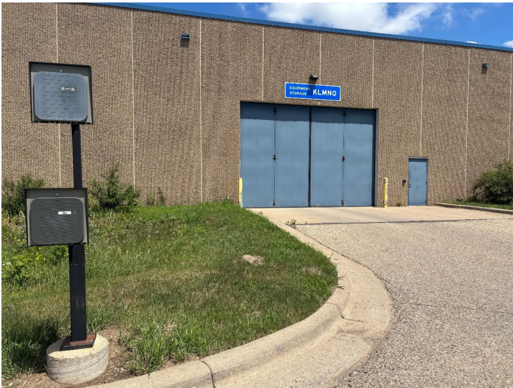
Figure 6 - Southeast Exterior Door View
