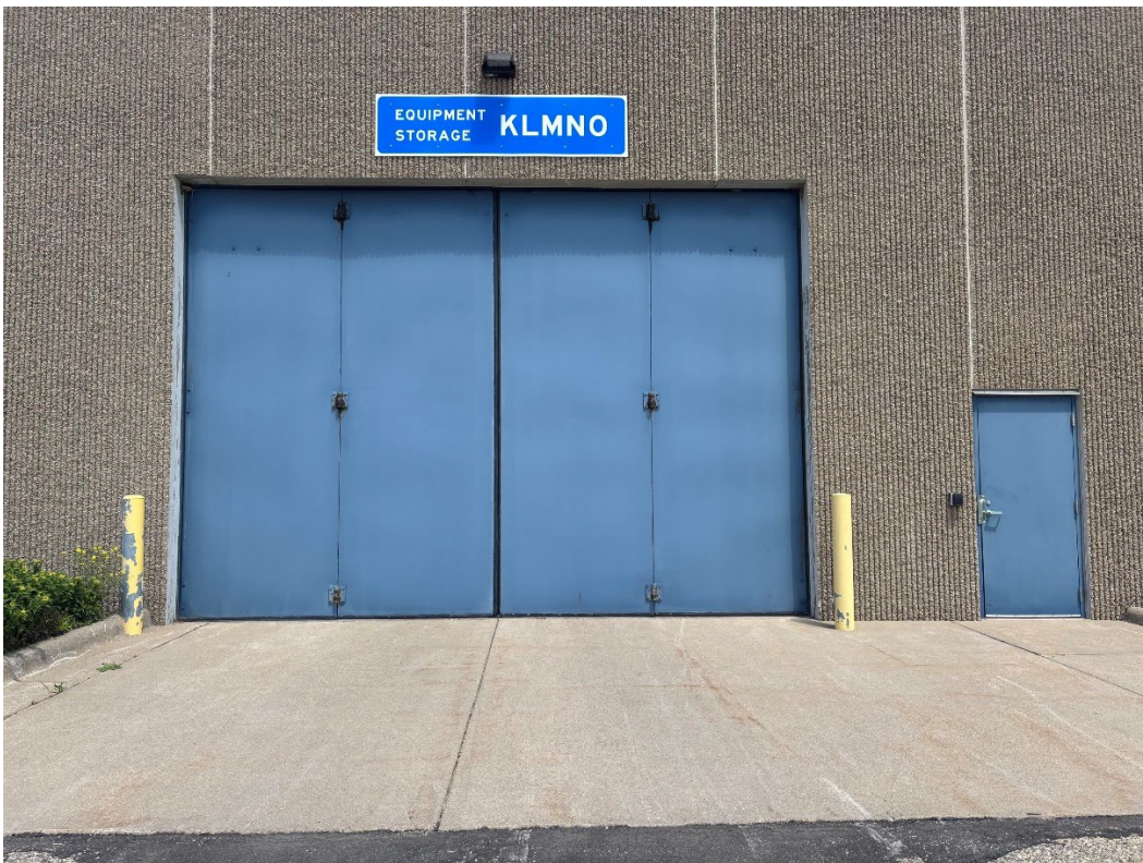
Figure 4 - Southwest Exterior Door View
